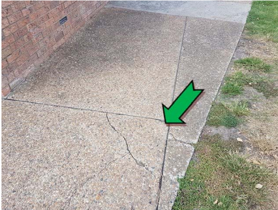
Photo 1. Exterior, ground, throughout, expansion joint – non asbestos-containing construction joint mastic.
